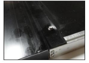
■Step 5: Do not over tighten the screws. Doing so may crack or damage the vinyl throwers. To ensure the proper installation of the vinyl throwers, we recommend that you install a wall vent into the house before installing the rest of your throwers. If you have questions, please contact us at 870-878-6805.
