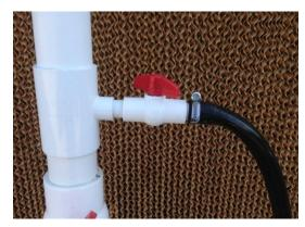
The desired setting should be determined during commissioning by "calibration": With the system running, set the  $\frac{1}{2}$ " ball valve so that, e.g., a 5-liter bucket can be filled in 20 seconds.
